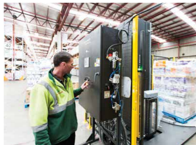
Countdown Distribution Palmerston North
